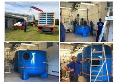
On site assembling
