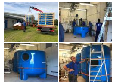
On site assembling
